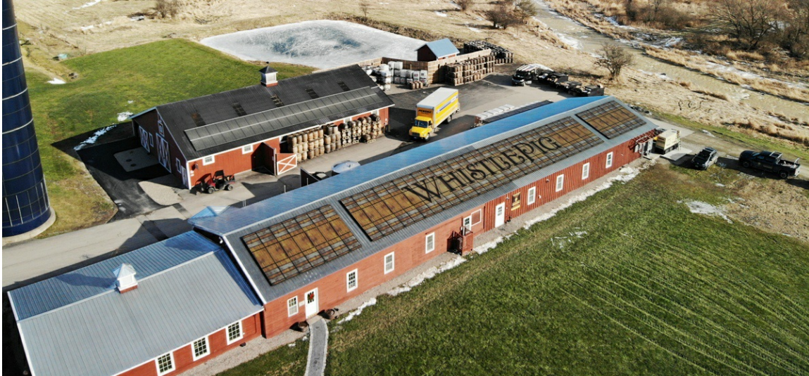
WhistlePig Whiskey Solar Array across the distiller's warehouse building and bottling plant Courtesy of Andrew Braden, WhistlePig
